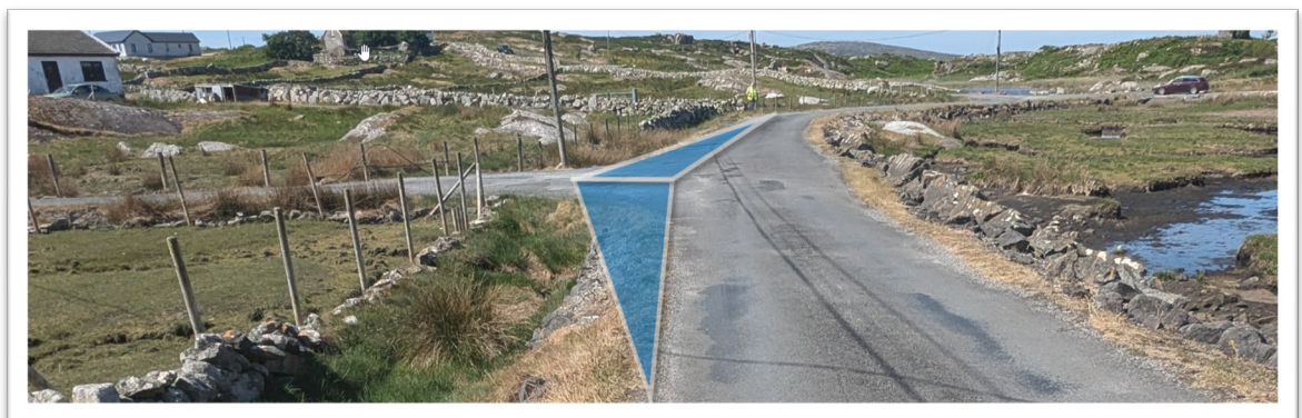
Figure 2.2 – Example Side Road B – Junction Sight Lines Which Should Be Maintained
